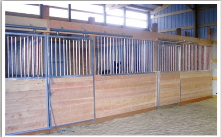
Solid welded grille 1-piece sections
