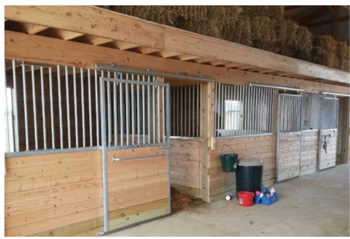
Solid welded door frame
